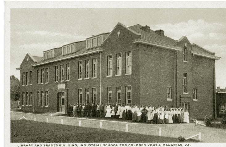
LIBRARY AND TRADES BUILDING, INDUSTRIAL SCHOOL FOR COLORED YOUTH, MANASSAS, VA.
